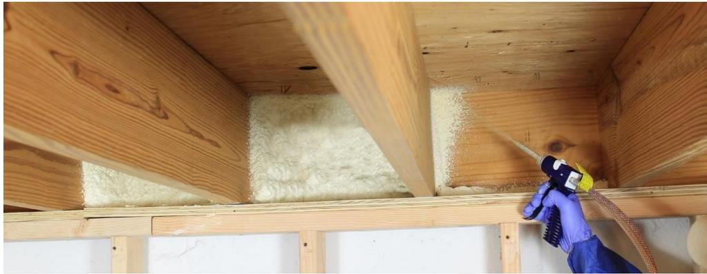
Spray foam hides, provides protection, and enables termites to move undetected to find and exploit food sources.
